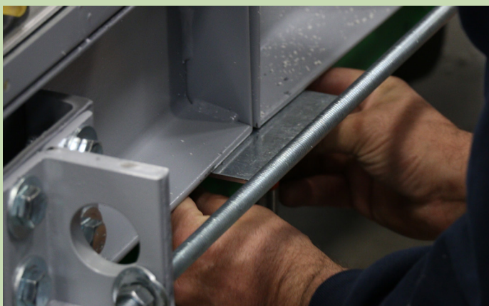
Adding shims to shore up unit
