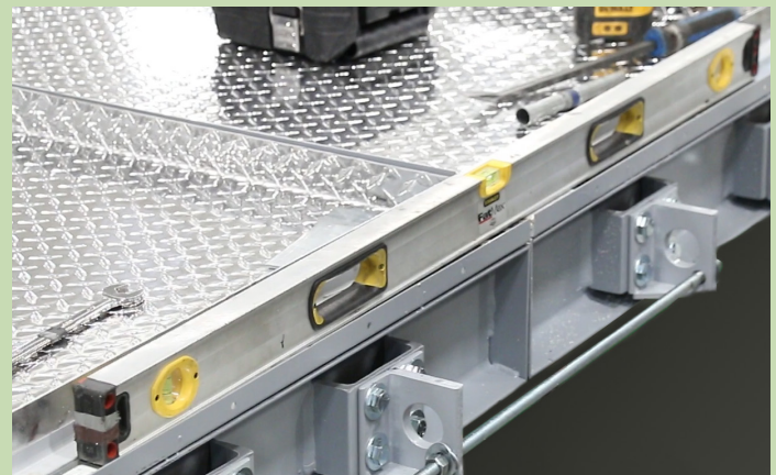
Using level to adjust base
