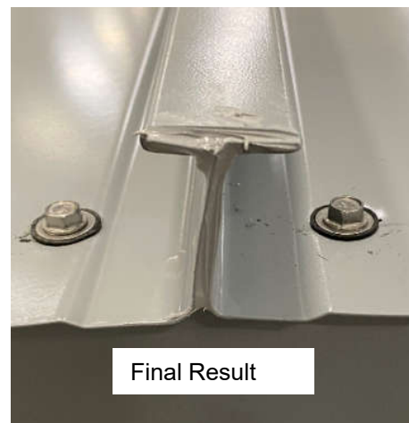
Detail 6 - Modular Third Liner Cap Installation using tool (Outdoor unit only)
