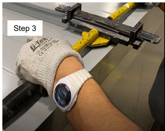
Detail 6 - Modular Third Liner Cap Installation using tool (Outdoor unit only)
