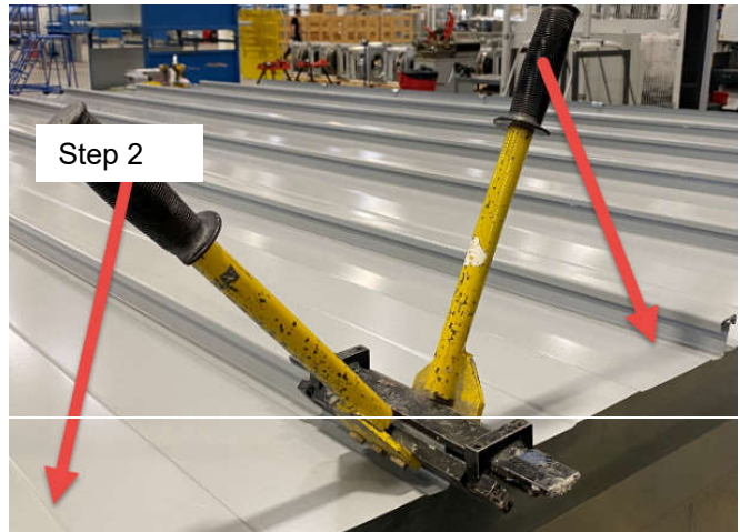
Detail 5 - Modular roof third liner detail (exterior Unit Only)
